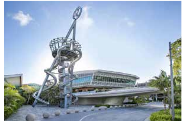
Aventura Mall Expansion III
